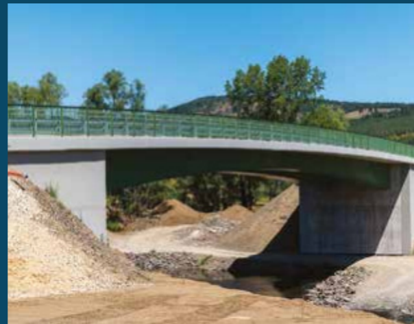
Ipolydamásd Ipoly-híd Bridge over the Ipoly at Ipolydamásd
